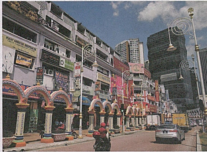
The 4 1/2-storey shops along Jalan Tun Sambanthan.
